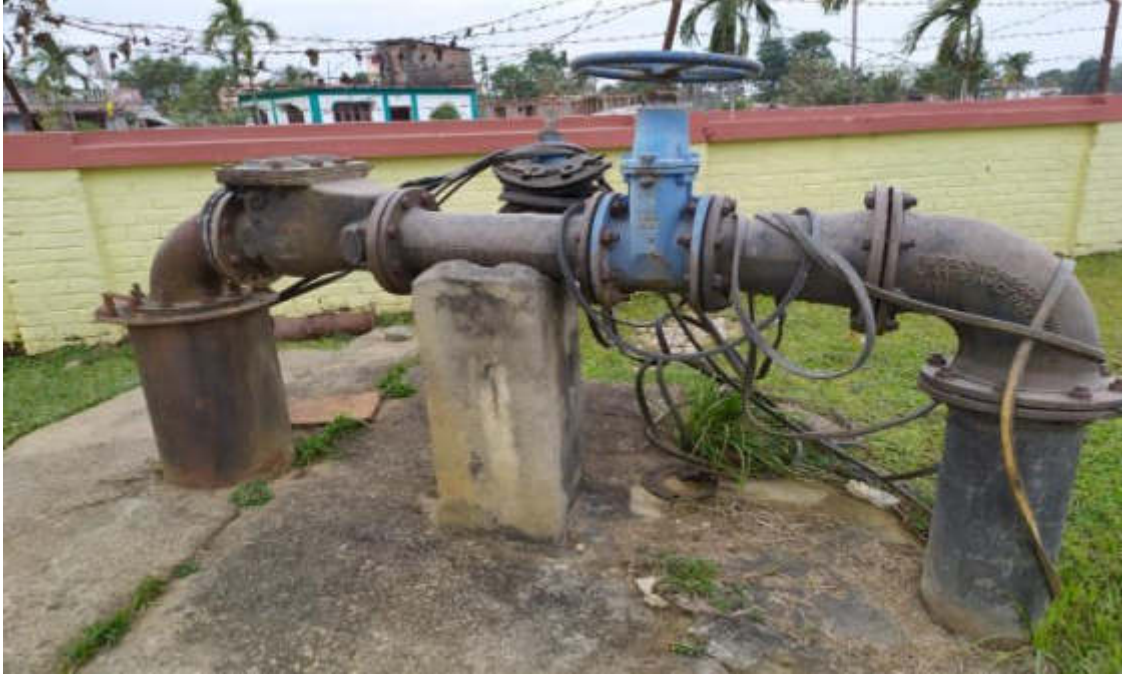
Bore Hole, OHT-2, Arjun Dhara Municipality-6, Birtamod
