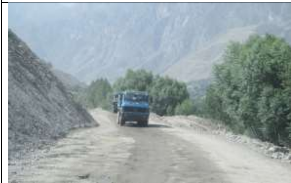
Water spraying at km 34+700
