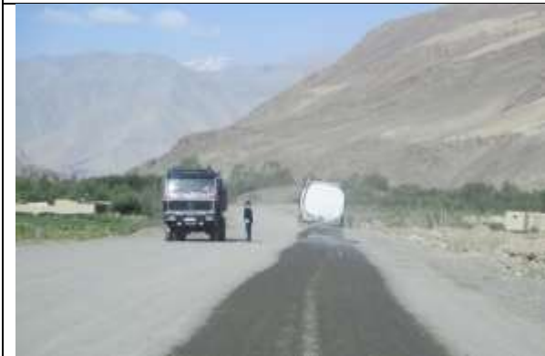
water spraying at km 29+600
