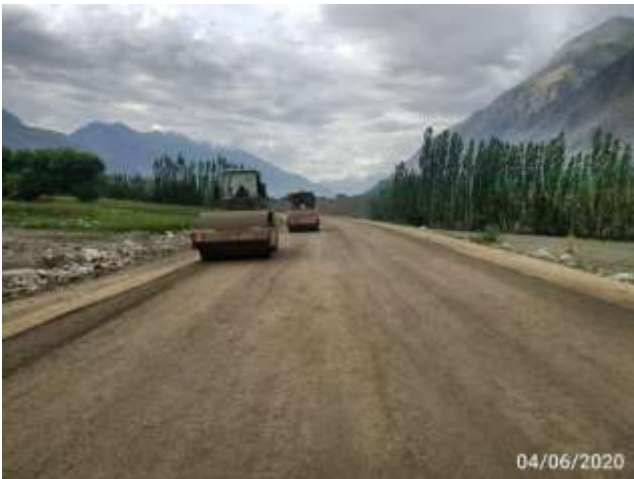
Compaction of the Subgrade at km 22+300
