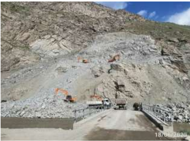
Hard cutting at km 32+500
