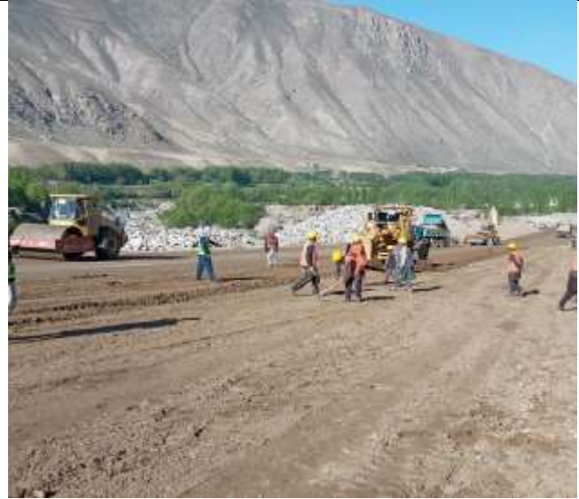
Subgrade compaction at km36+900
