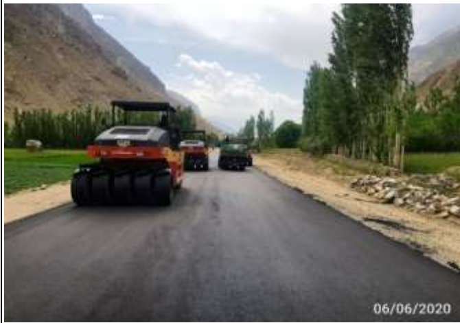
Binder work at km 7+600
