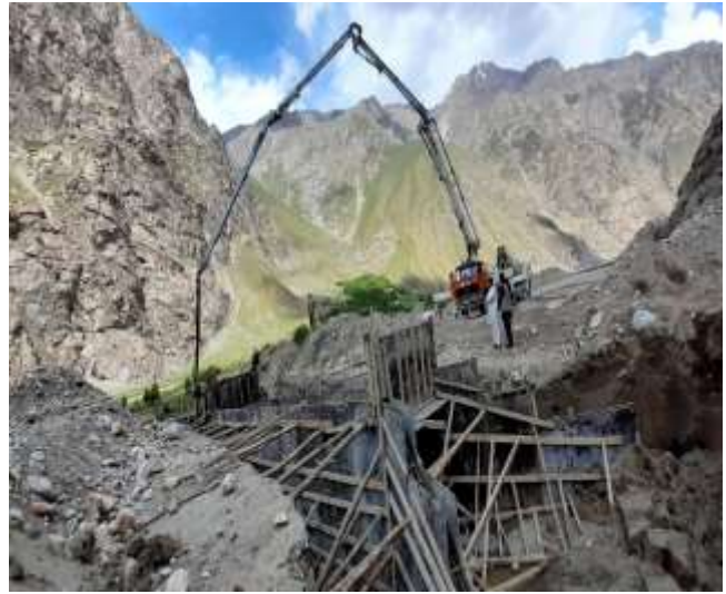
Puring of the concrete of box culvert at km 16+500
