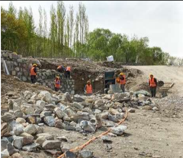
Raitining wall at km 17+700
