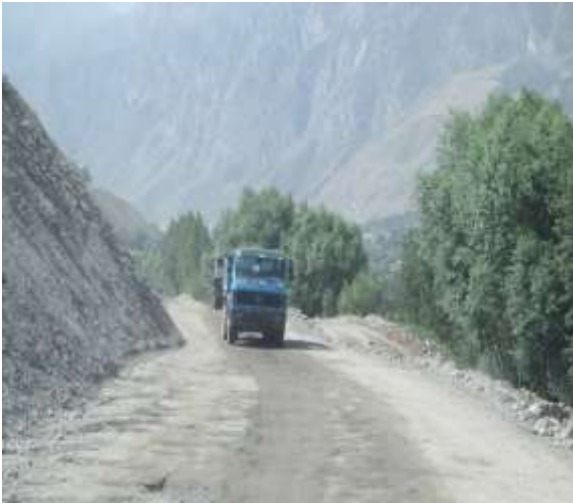
Water spraying for the control of dust at km 5+300
