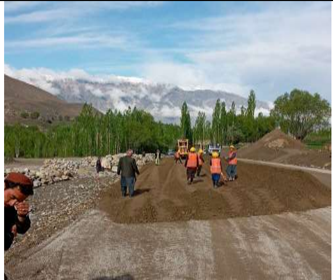
Sub base at km 77+900
