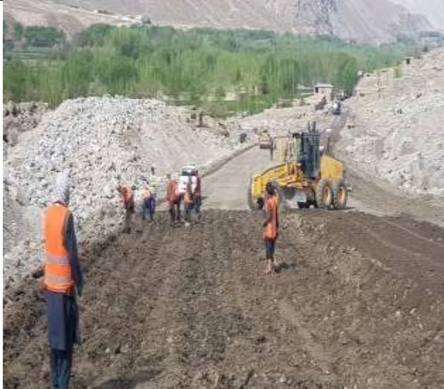
Subgrade preparation at km 4+600
