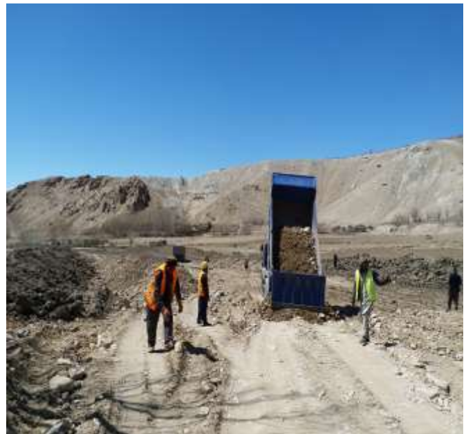
Construction at km 44+700
