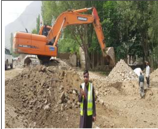
Noise level at constrction site km 33+400
