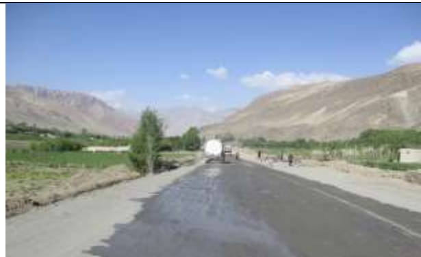
water spraying at km 29+300
