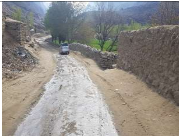
Water spraying at km 3+400
