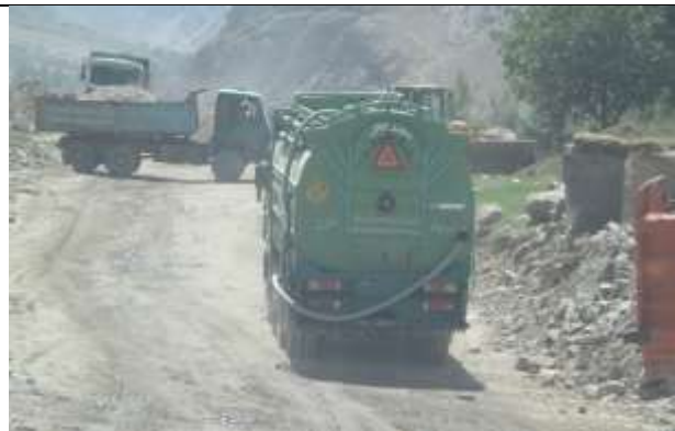
Water spraying at km 77+100
