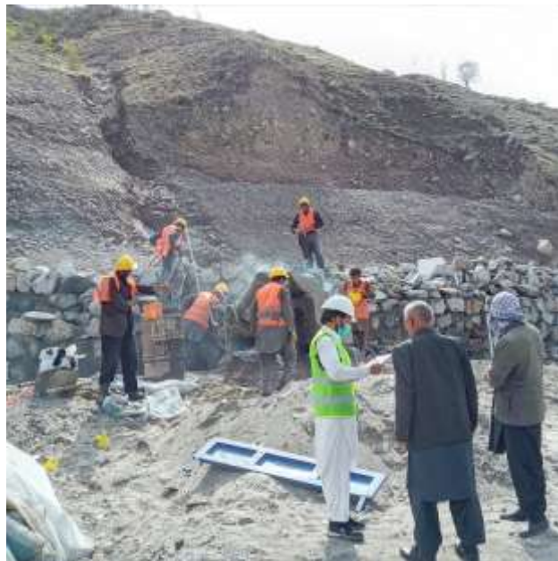
Retining at site km 66+600
