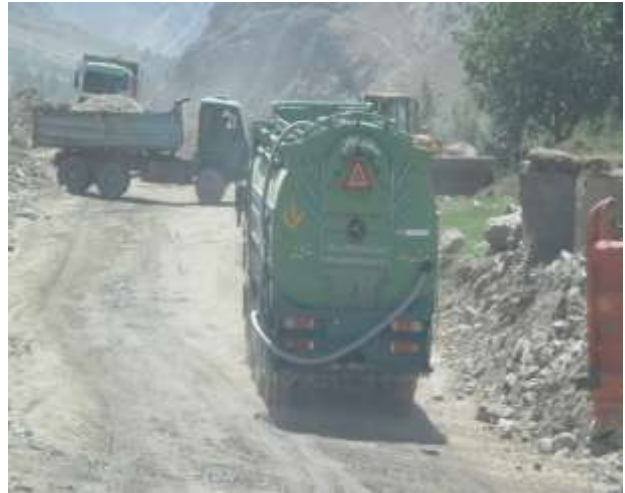
Water spraying for the control of dust at km 12+300
