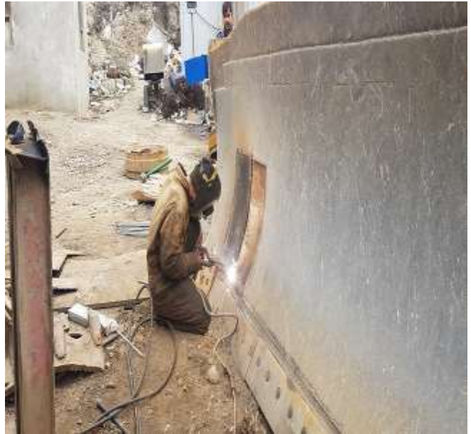
Welding work at workshop km 70+900
