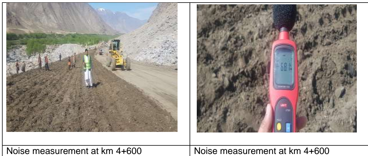
Figure 5: Noise level measurement at different location
