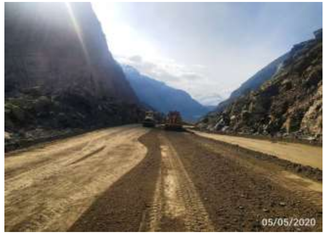
Compaction of the Subgrade at km 66+330
