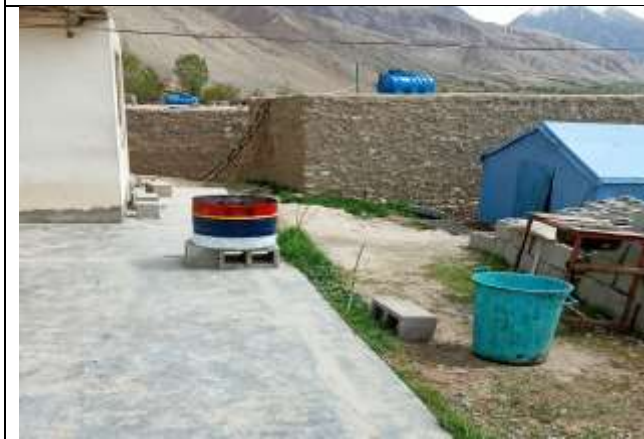
Waste collection system at contractor office km 13+300
