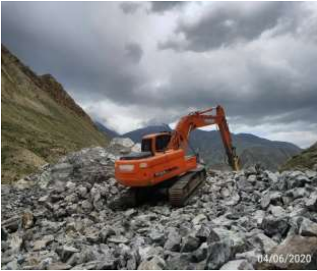
Hard cutting at km 33+400
