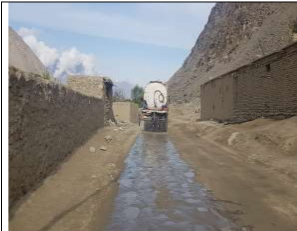
Water spraying at km 2+900
