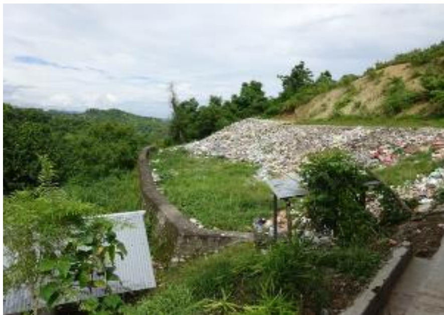
Photograph 1: Present solid waste landfill site
