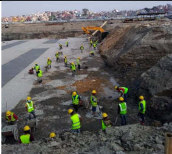
Figure: PPEs worn by worker of TP03
