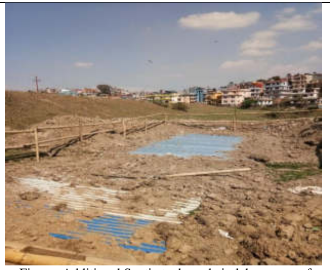
Figure: Additional Septic tank made in labor camp of TP03.
