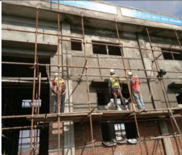
Figure: Workers provided with harness during work at height (TP-02)
