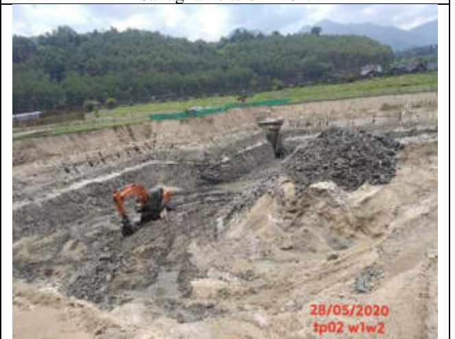
Figure: Benching method applied in excavation in TP02
