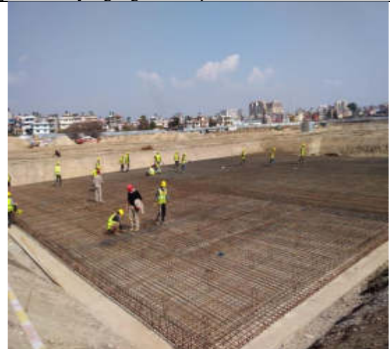
Figure: Sloping method used while excavating in TP03
