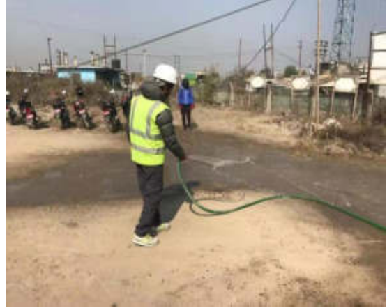
Figure: Water is being sprayed in TP02 for dust suppression
