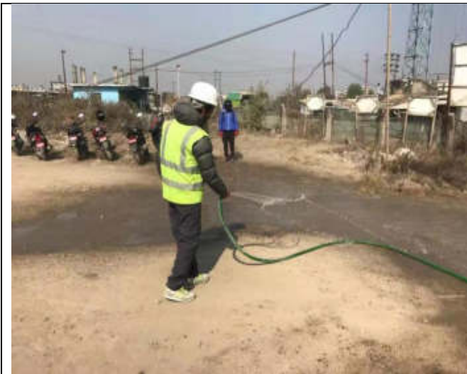
Figure: Water is being sprayed in TP02 for dust suppression.
