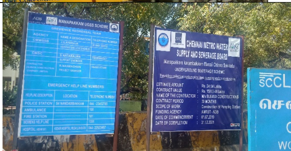
CMWSSB-UGSS – GRM & Project info Disclosure at worksite
