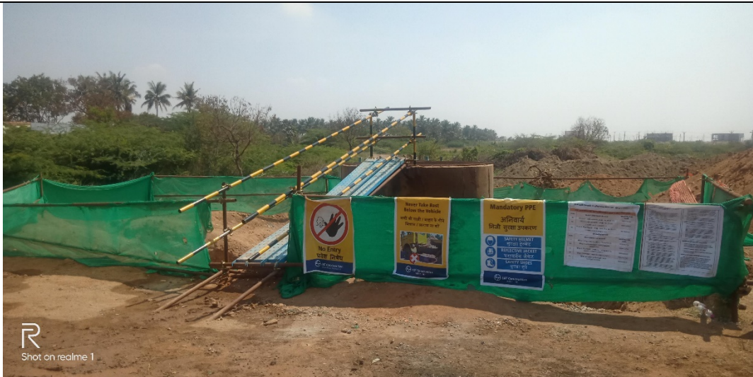
Coimbatore UGSS – Lift station works with safety measures
