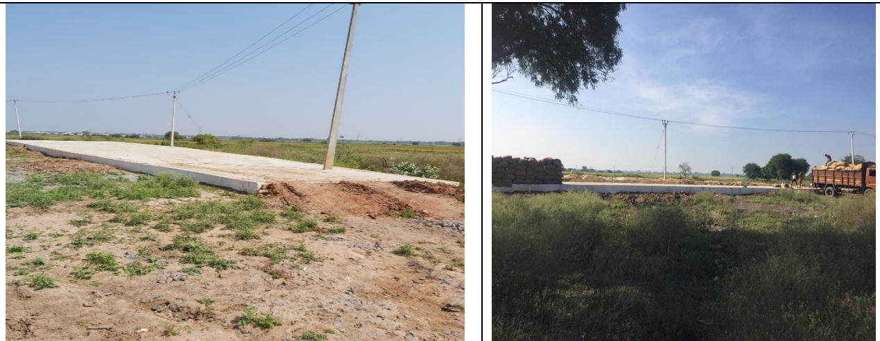
Trichy UGSS – Phase -II New Agriculture threshing platform
