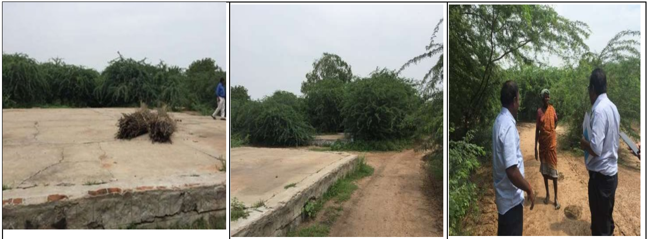
Trichy UGSS-Phase-II - Old Agriculture threshing platform
