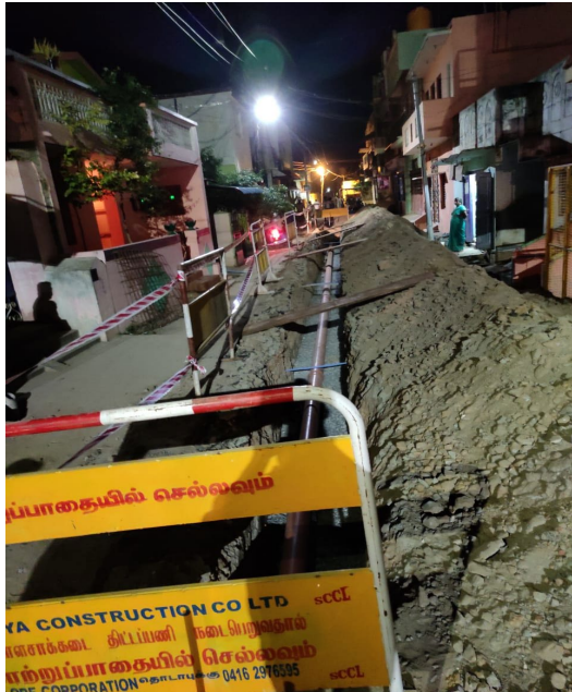
Vellore UGSS – Phase II Works
