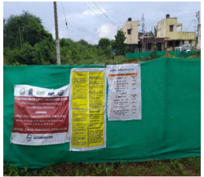
Disclosure of GRM in project site – Coimbatore UGSS
