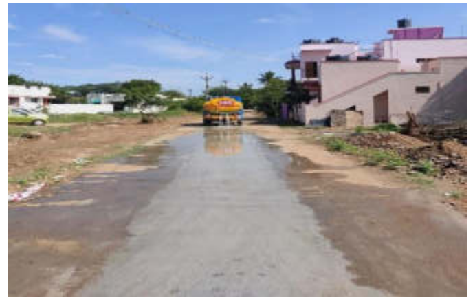
Road restoration in progress – Coimbatore UGSS Package 1
