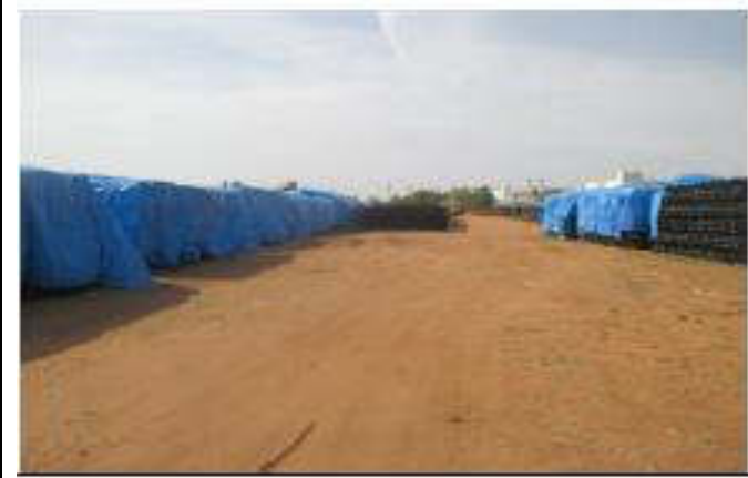
Material Storage - Tirunelveli UGSS Ph-III
