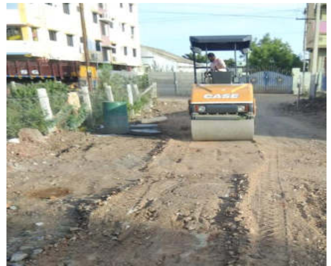
Road Compaction in progress - Trichy UGSS Package 2
