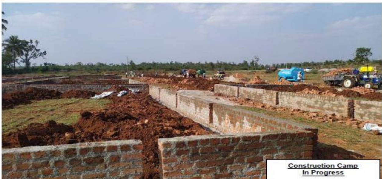
ESTABLISHMENTS OF THE CONSTRUCTION SITE AND PLANT SITE ITAGI CAMP, KM 161+700
